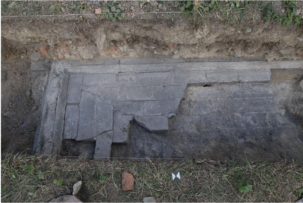
Picture 14. Part of the preserved washroom / laundry floor with visible concrete foundations.
